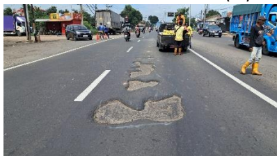
JALAN LINGKAR WELERI KM 47+800 (0%)
