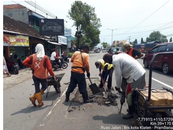
PENANGANAN LUBANG BTS KOTA KLATEN-PRAMBANAN (BTS. DIY) KM. 39+170 KI
