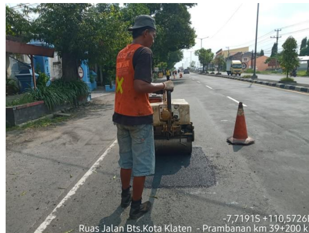
PENANGANAN LUBANG BTS KOTA KLATEN-PRAMBANAN (BTS. DIY) KM. 39+200 KI
