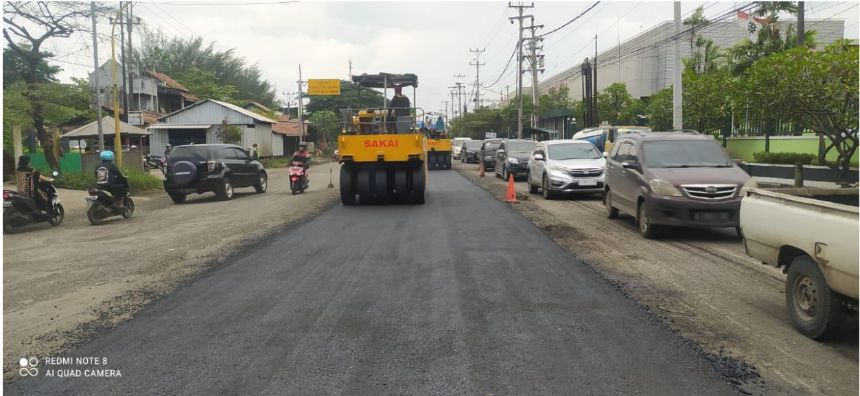
Rehabilitasi mayor ruas Kudus – Pati KM 62 (4/3/2023)
